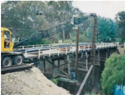
Above: 310UC97 steel piles driven from the riverbank.
